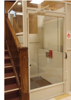
One of the new wheelchair lifts providing greater accessibility to TimeLine's Wellington Avenue theatre space.
