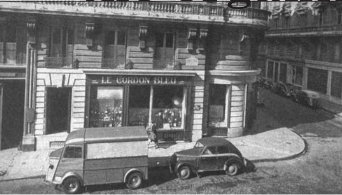
Exterior of Le Cordon Bleu in Paris.
